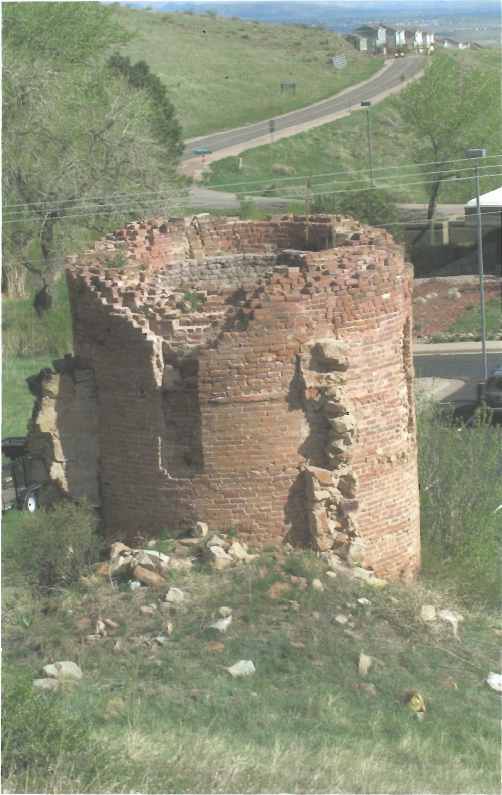
14. Remains of the Silica lime kiln at the site of the Silicated Brick Company- May, 2006 View looking northwest showing the internal structure of the kiln.
