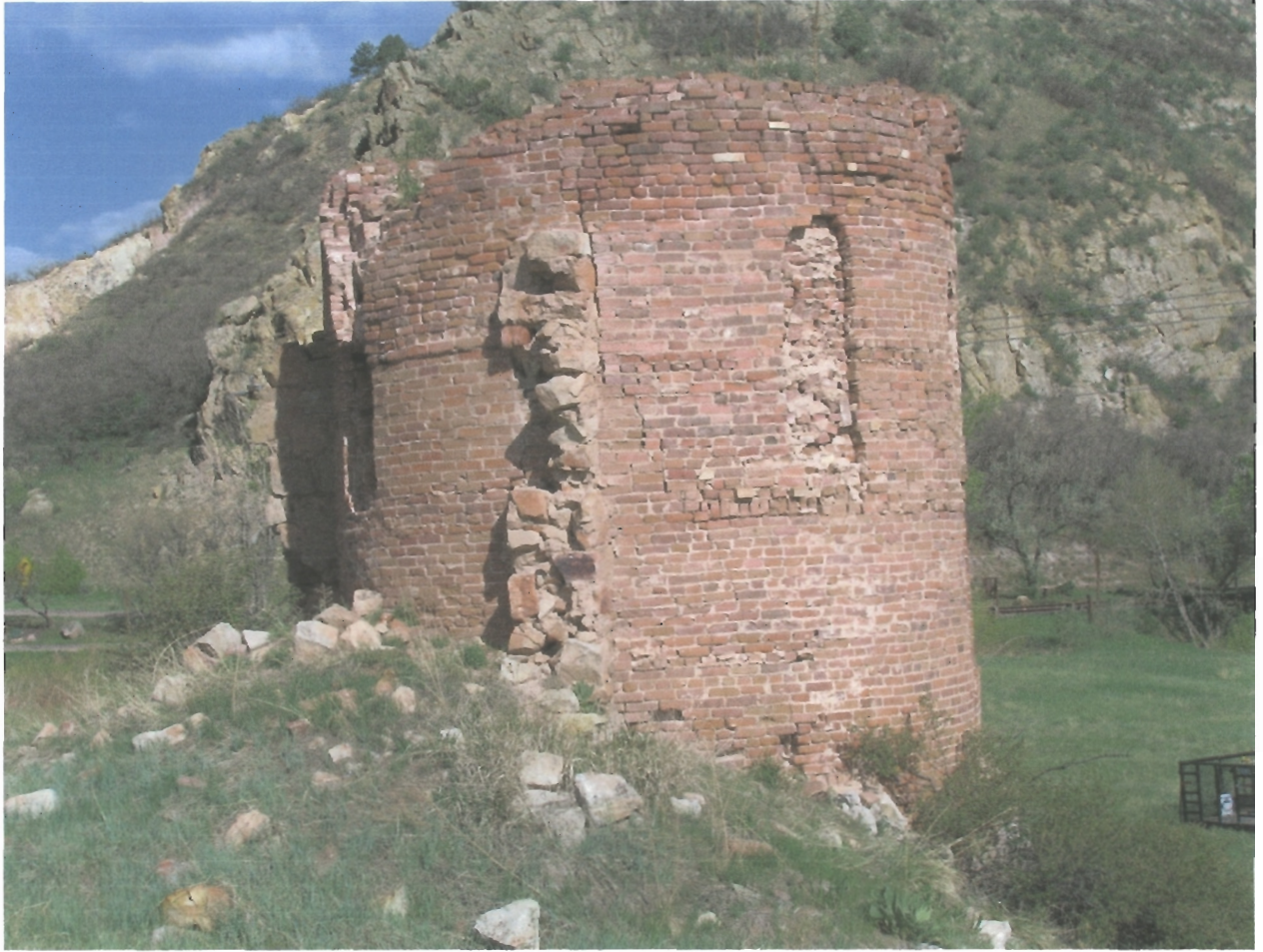
12. Remains of the Silica lime kiln at the site of the Silicated Brick Company- May, 2006 View looking west
