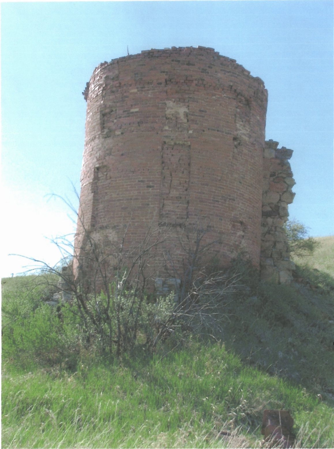
11. Remains of the Silica lime kiln at the site of the Silicated Brick Company- May, 2006 View looking southeast
